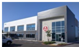
AGC East County Facility & Apprenticeship Training Center
