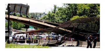
On June 23, a truck struck the low clearance Lane Pace Pedestrian Bridge spanning Interstate 295 in Washington, D.C., causing it to collapse and injure five people. The collapse tangled traffic for 12 hours. In the bridge's most recent inspection prior to the collapse, it had been deemed to be in poor condition and failed to meet height requirements.
